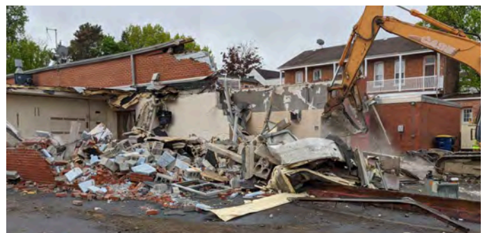
The old Station 1 being demolished in early 2020.
